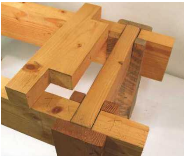
▲ Pic.11 End rail removed to show construction
